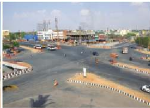
PVN Express Flyover joining Junction
