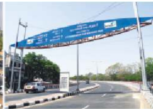
Entrance of PVN Express Flyover
